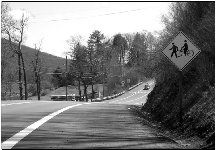
Wide shoulders and signage for bicycle/pedestrian use along US 219. Note the marked crosswalk in the background.
